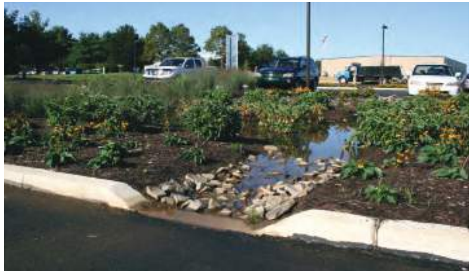
Streetscaping can integrate stormwater management features such as bioswales or rain gardens.
